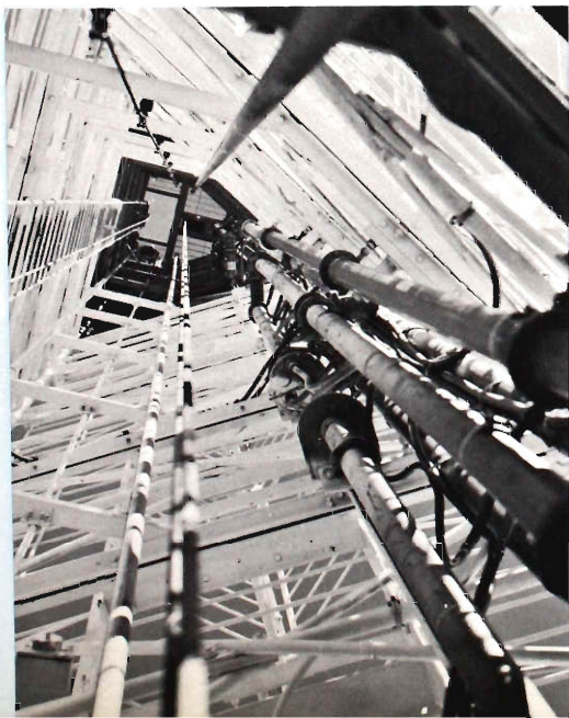
FIG. 5 (lower left) Another view from service elevator, inside tower, showing part of antenna feed system and junction box.
